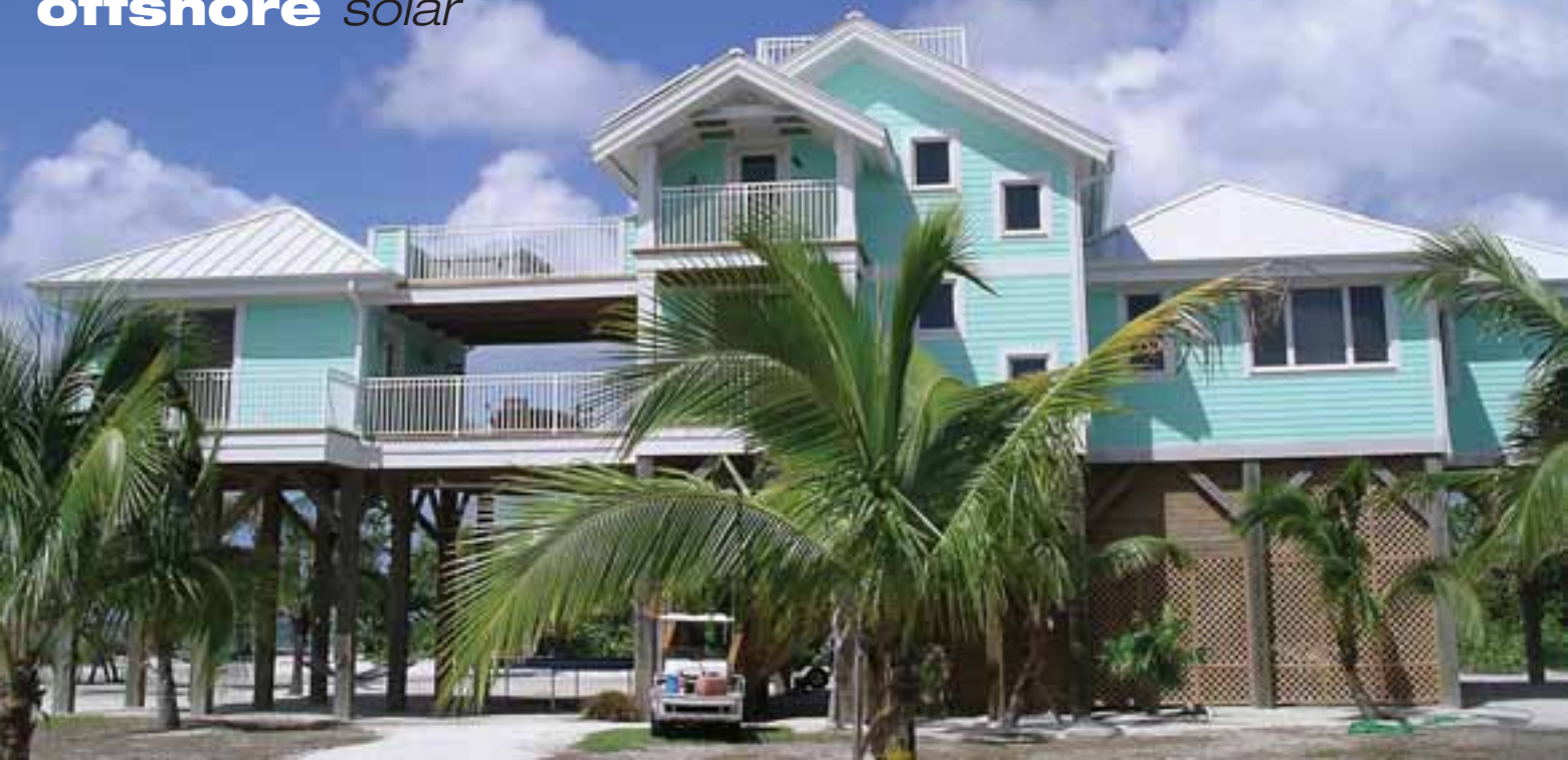
Elevated to second-story level, the McVickers' house is designed to catch cool ocean breezes. Deep roof overhangs shade the windows and help their home keep cool.
