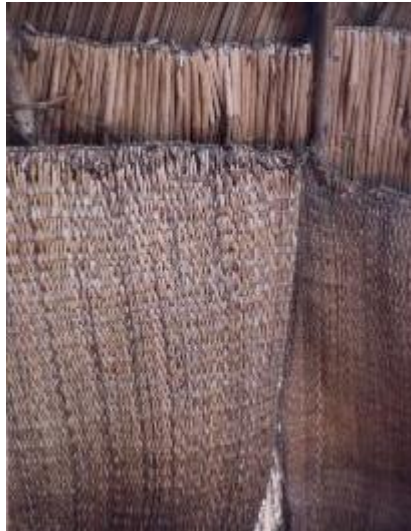
WOVEN INTERIOR MATS ON BOTTOM WITH SEWN EXTERIOR MATS SHOWING BEHIND ON TOP FROM A WIGWAM AT PLIMOTH PLANTATION.
