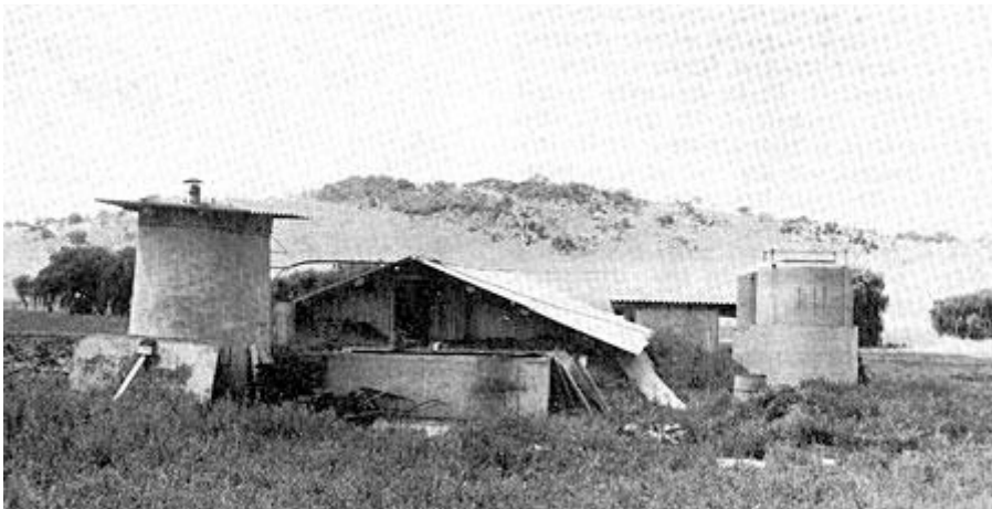
Fig. 32 Digester with storage tank in background
