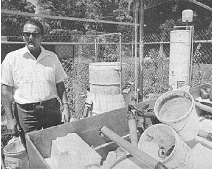
Mr. L. John Fry beside a three-digester unit he made in 1973. Gas holder center, water-heater on the right. Buckets in the foreground were for loading raw materials. This unit was taken down in 1974.
