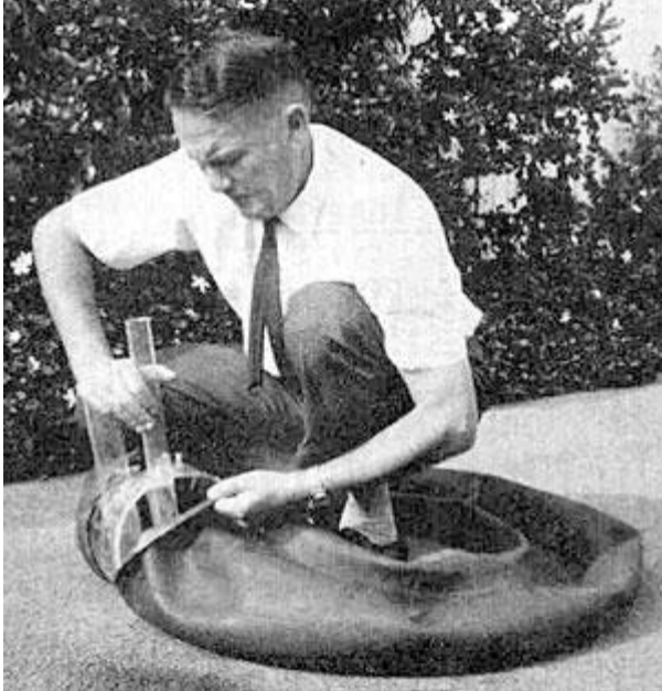
Fig. 25 Placing the cylinder in the inner tube
